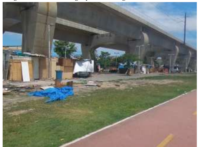
Figure 4: Parque Linear de Manguinhos (RJ): precarious and irregular buildings and housing (Photo by Danielle Carvalho, 2017)
